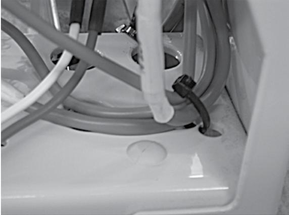
***Figure D-9: Cables secured to frame with tie***
